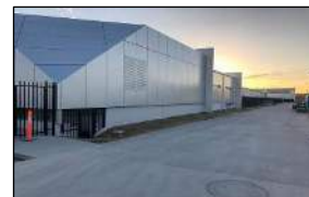
I Seek Data Centre Brisbane Airport
